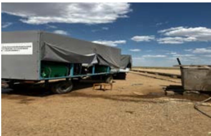
Fig. 1 - Production tests of a mobile desalination plant in the Talas district of the Zhambyl region
